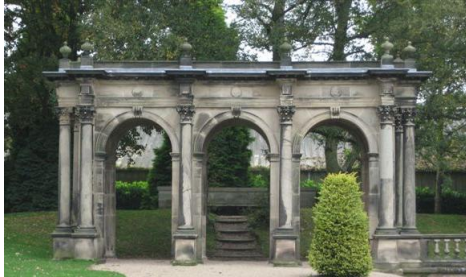
The last remaining loggia
